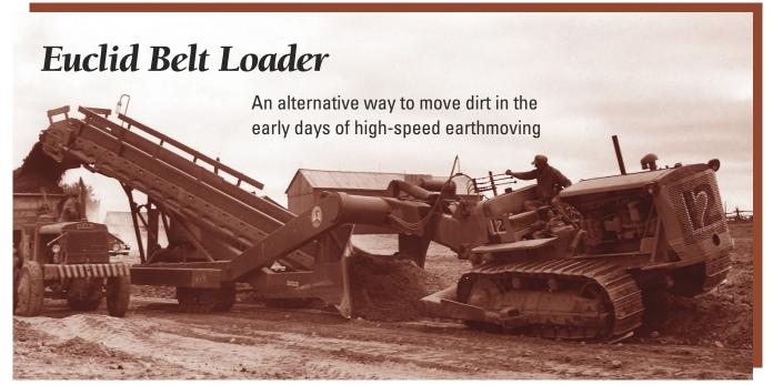
ust two years after LeTourneau introduced the first rubber-tired high-speed motor scraper in 1938, the Euclid Road Machinery Co. offered an alternative way of moving dirt at high speed over long distances.
